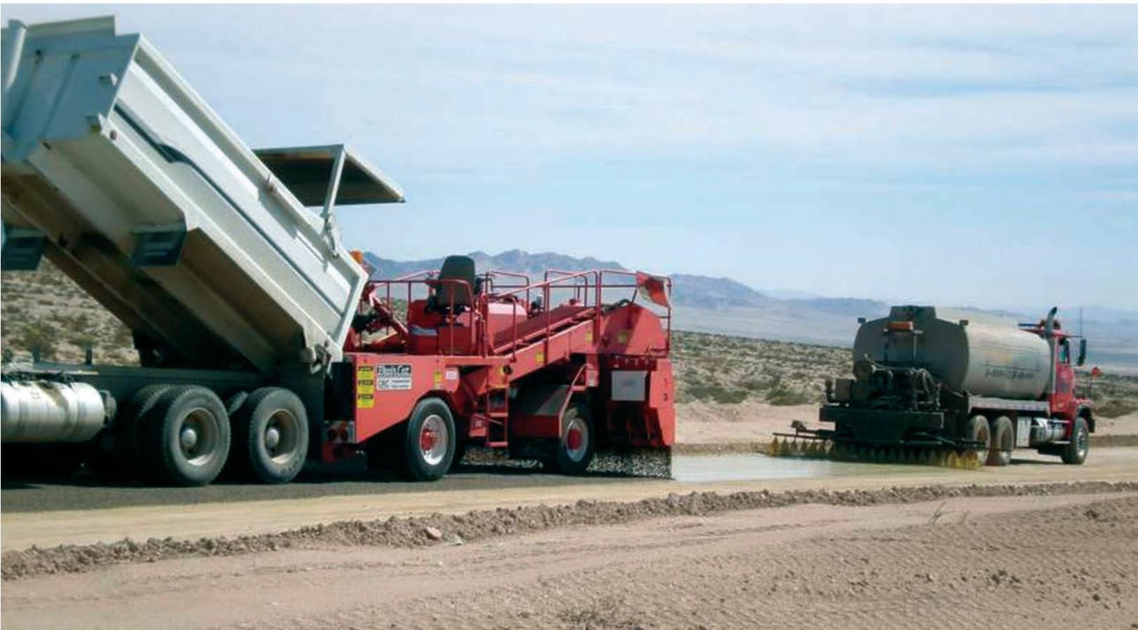
In some cases, a road has deteriorated to the point that a full-depth reclamation is required. If this is the case with your road, Midwest offers stabilization solutions that are less invasive and costly than traditional methods. And in doing so, we can increase the California Bearing Ratio (CBR) of your road by 80% in just 48 hours.
