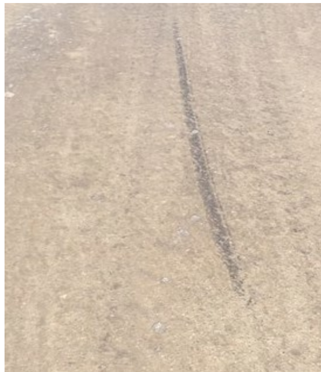
East Road – surface
