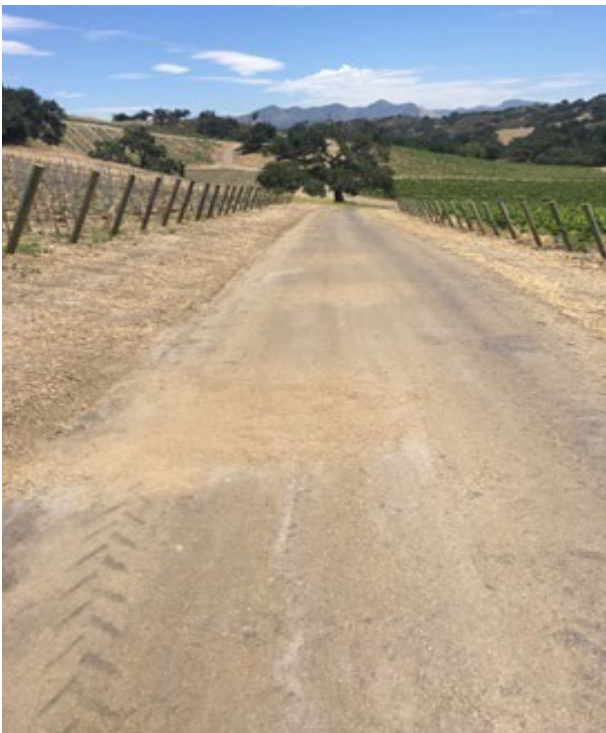
North Road- repair area
