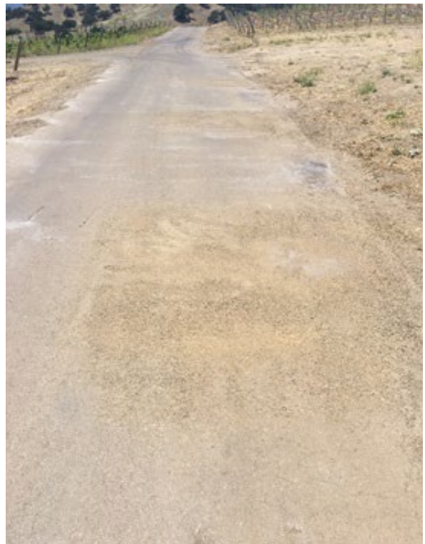
North Road- repair area
