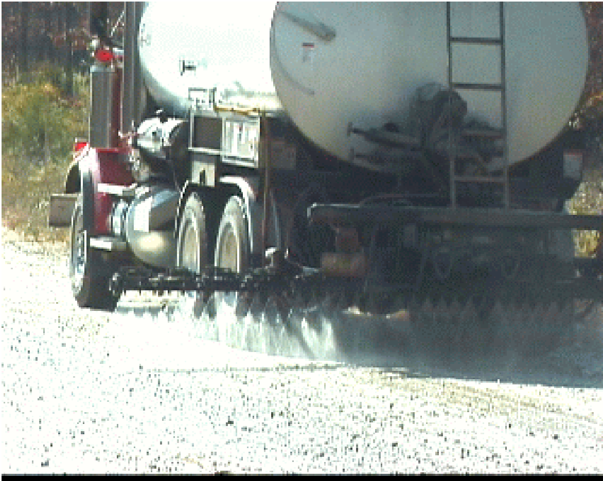
Figure 3. Application of EnviroKleen®
